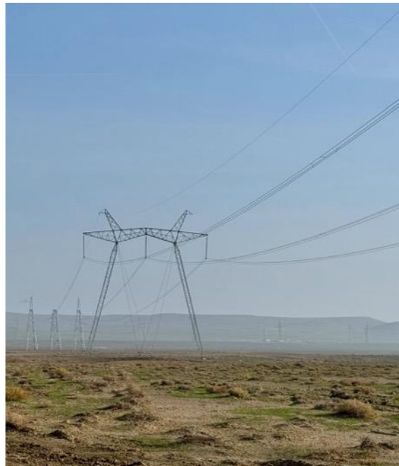
Newly installed OHL towers at Absheron-Garadagh, going towards Navahi
